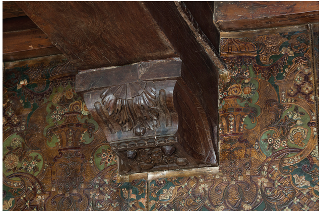
Fig. 19 Original consoles below the support beams. Photo: Cultural Heritage Agency of the Netherlands.
