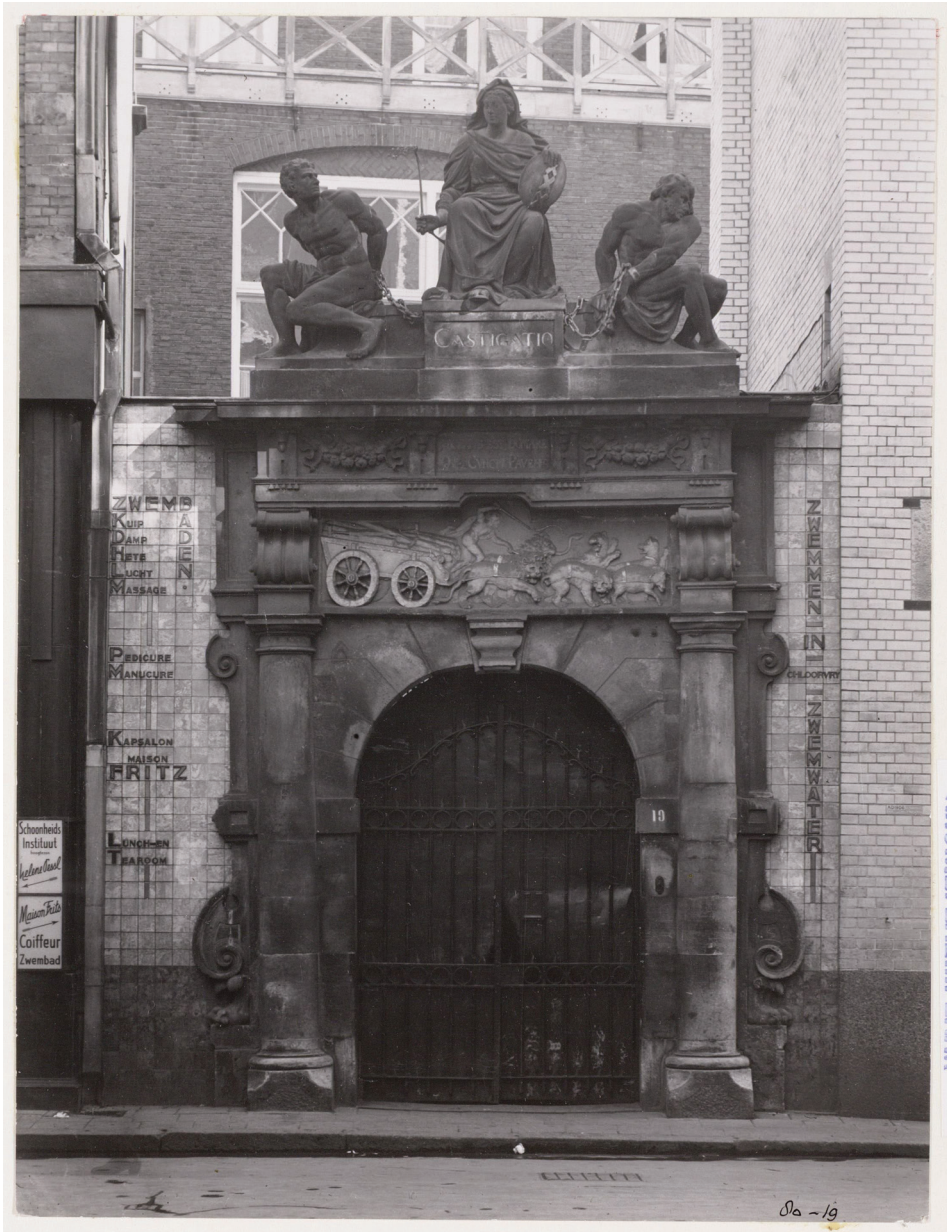
Fig. 9 Portal of the former Rasphuis at Heiligeweg 19, 1943, photograph, Amsterdam, Stadsarchief.
